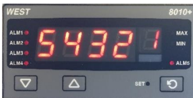
Photo shows all alarms active and the Alarm Status.
